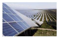
Solar photovoltaic panels (solar PVs) can be installed on individual buildings or housings but can also be created as community solar PVs. In the case of community solar PVs, large land areas are required in order to install this renewable energy power source. Also called solar farms, approximately 100 square feet of land is required for every 1kW of solar panels for a typical installation.
